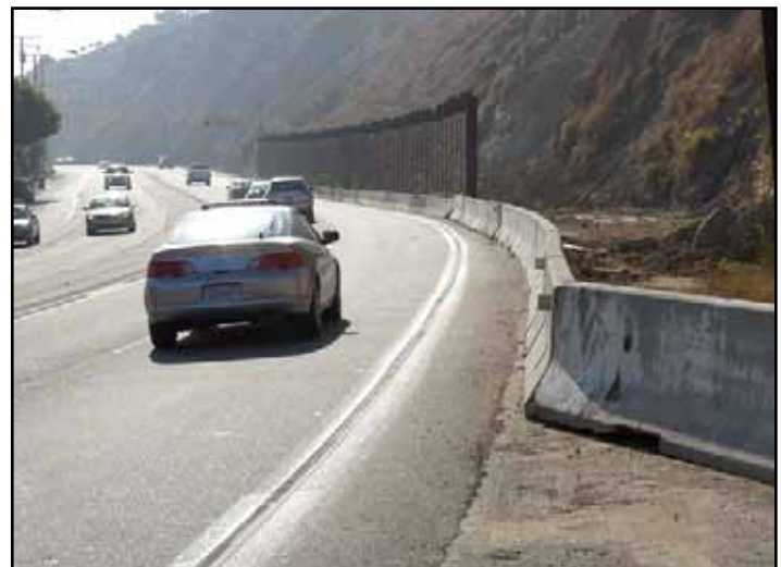
Slide barrier, South of Malibu. This barrier will be there forever.
