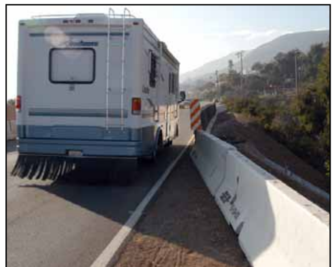
Bridge construction, just North of Trancas
